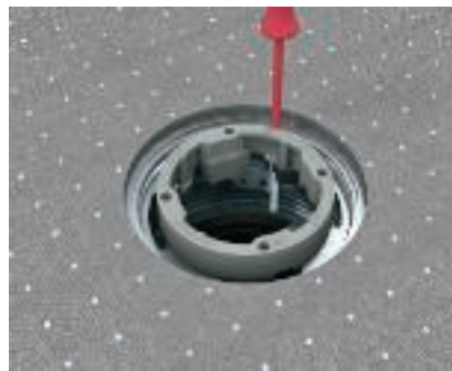
Telitank mounting on underfloor outlet US80 and underfloor box UDL2-80 Turn the internal mounting ring into the top area of the outlet and secure it by turning in the clamping screw. The inserted spacer ring should be roughly flushed with the top edge of the finished floor.
